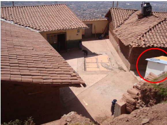
August 2012 – The old bathrooms have been removed and the new bathrooms have been built in the corner of the patio. The Kindergaten has now been awarded the certificate they needed from the Defensa Civil of Peru. With this certificate, the Kindergaten now has an official license with their municipality.
